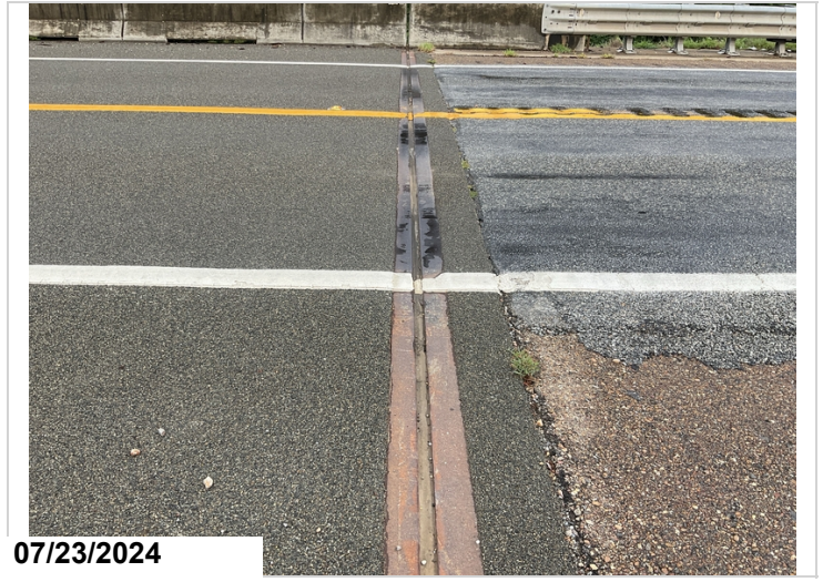
End of bridge joint
