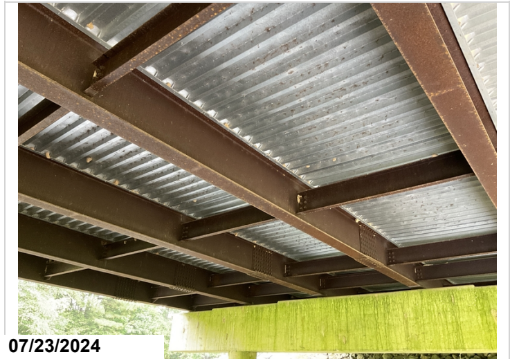
Weathering steel beams
