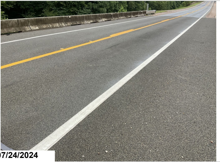
Deck, new polymer overlay
