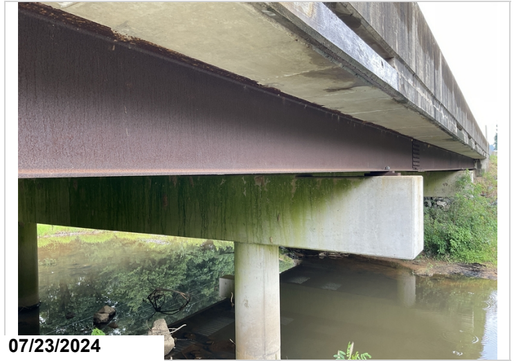
Continuous weathering steel beams
