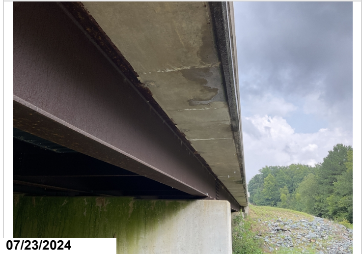
Various locations, Concrete deck overhangs, cracking with efflorescence, CS2.
