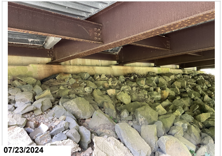
Bent 1 abutment, cracking with efflorescence, 4', CS2.
