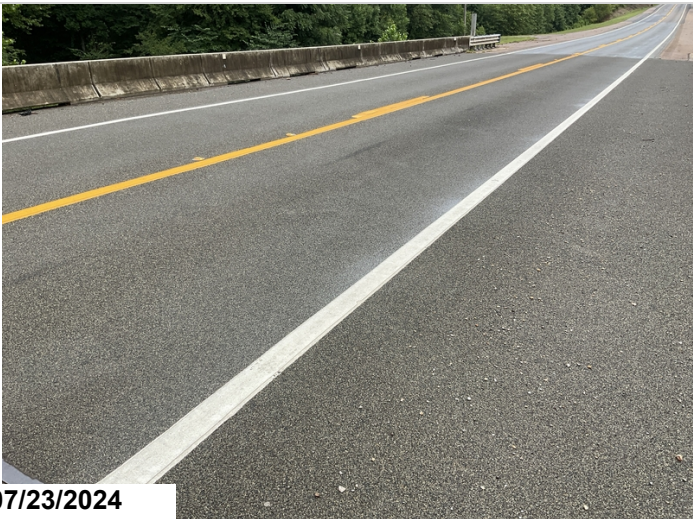
Deck, new polymer overlay
